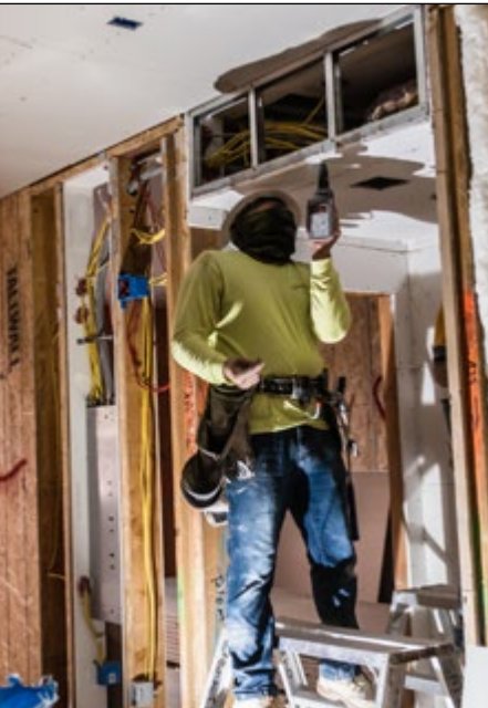
Drywall subcontractor installs 3/4" SOUND CURB on ceiling.
