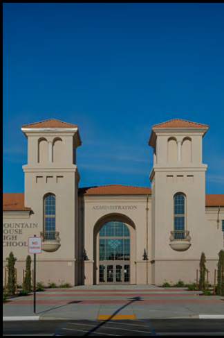
Just opened and now teeming with 400-450 underclassmen, the two-story classroom and administration building anchors the first-ever secondary school campus of the Lammersville, CA, Unified School District in Mountain House, CA.
